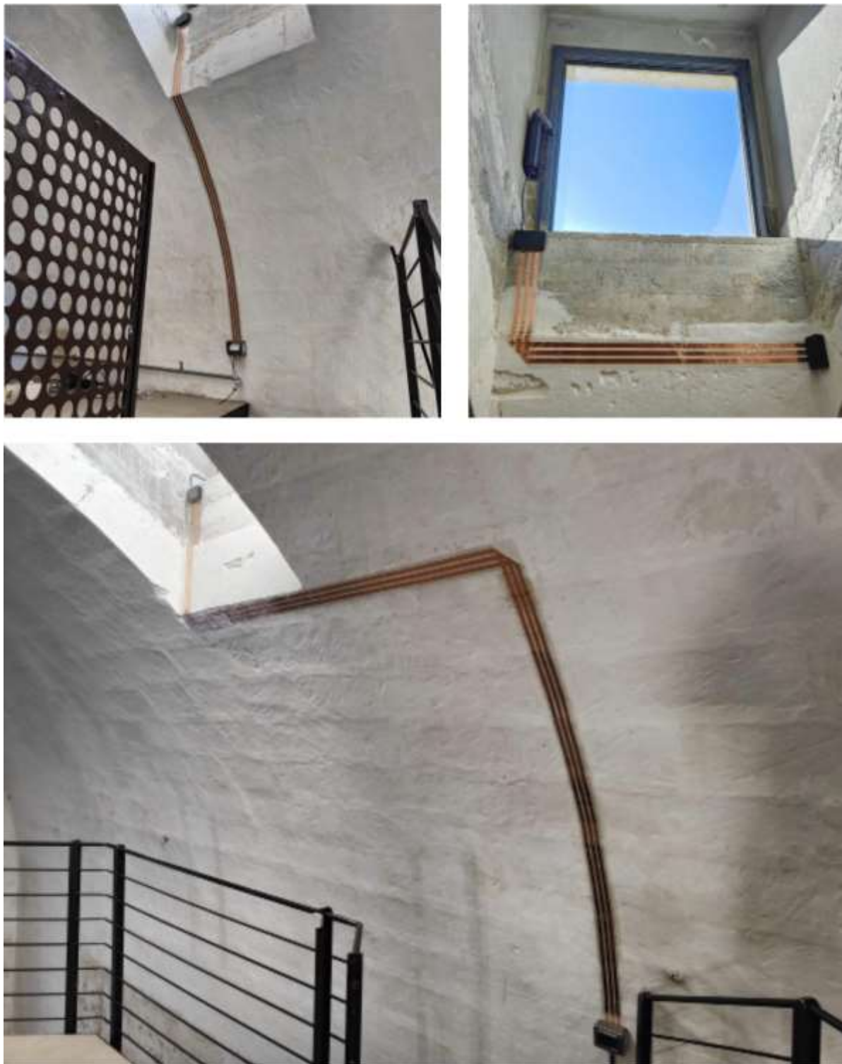
Figure 26: Construction of the electrification system of a skylight with Next-Tape NM3BT15 for a vaulted room in Matera
