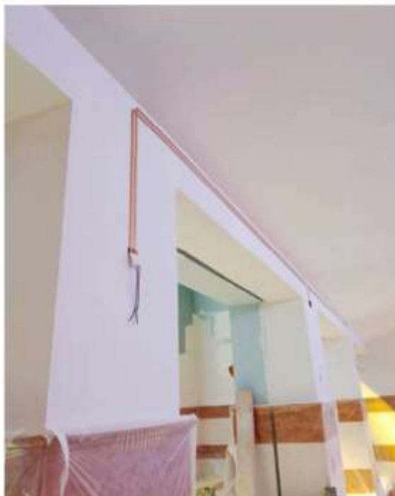
Figure 24: Implementation of a lighting system using NM3BT15 electrical tape in a church in Andria, Apulia, Italy.
