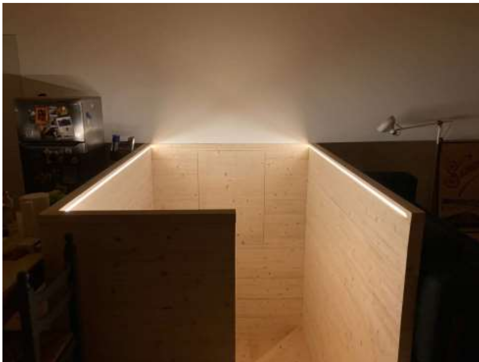
Figures 41: An example of installation of Next-Light on the upper edge of the interior staircase - Valdagno (Province of Vicenza).
