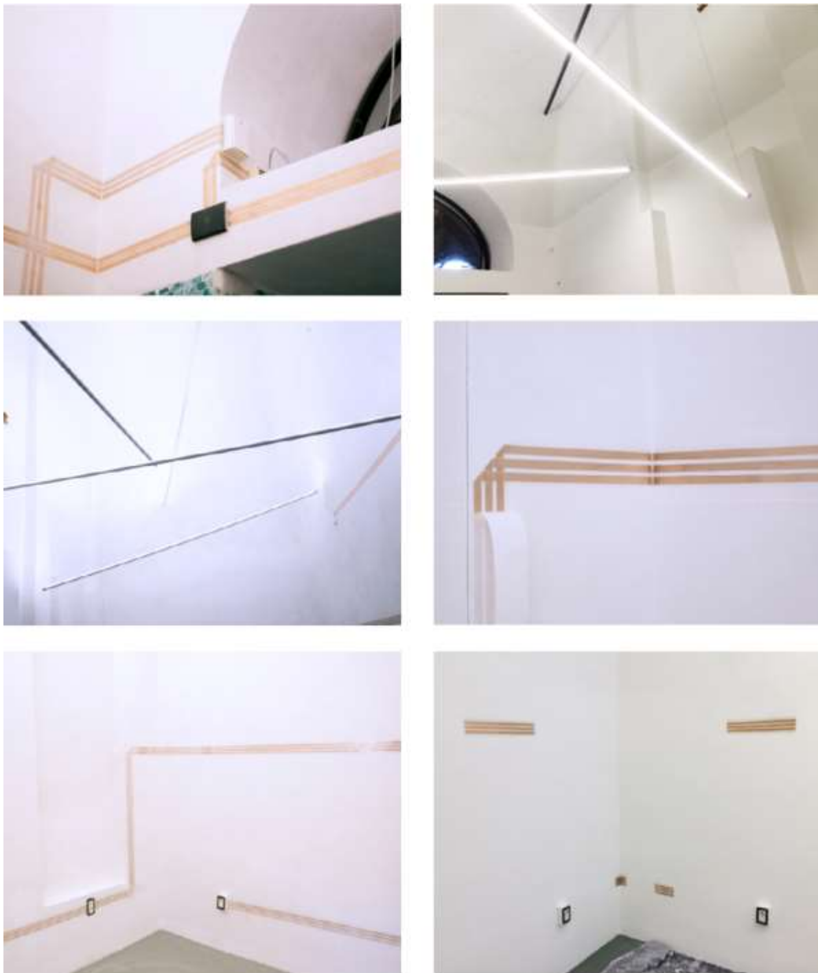
Figure 25: Implementation of the lighting system for "Under the Hall" at the Palace of Reason in Padua using NM3BT25 Electrical Tape and Next-Light LEDs.
