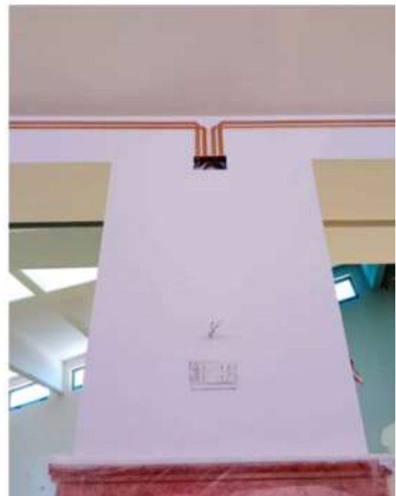
Figure 24: Implementation of a lighting system using NM3BT15 electrical tape in a church in Andria, Apulia, Italy.
