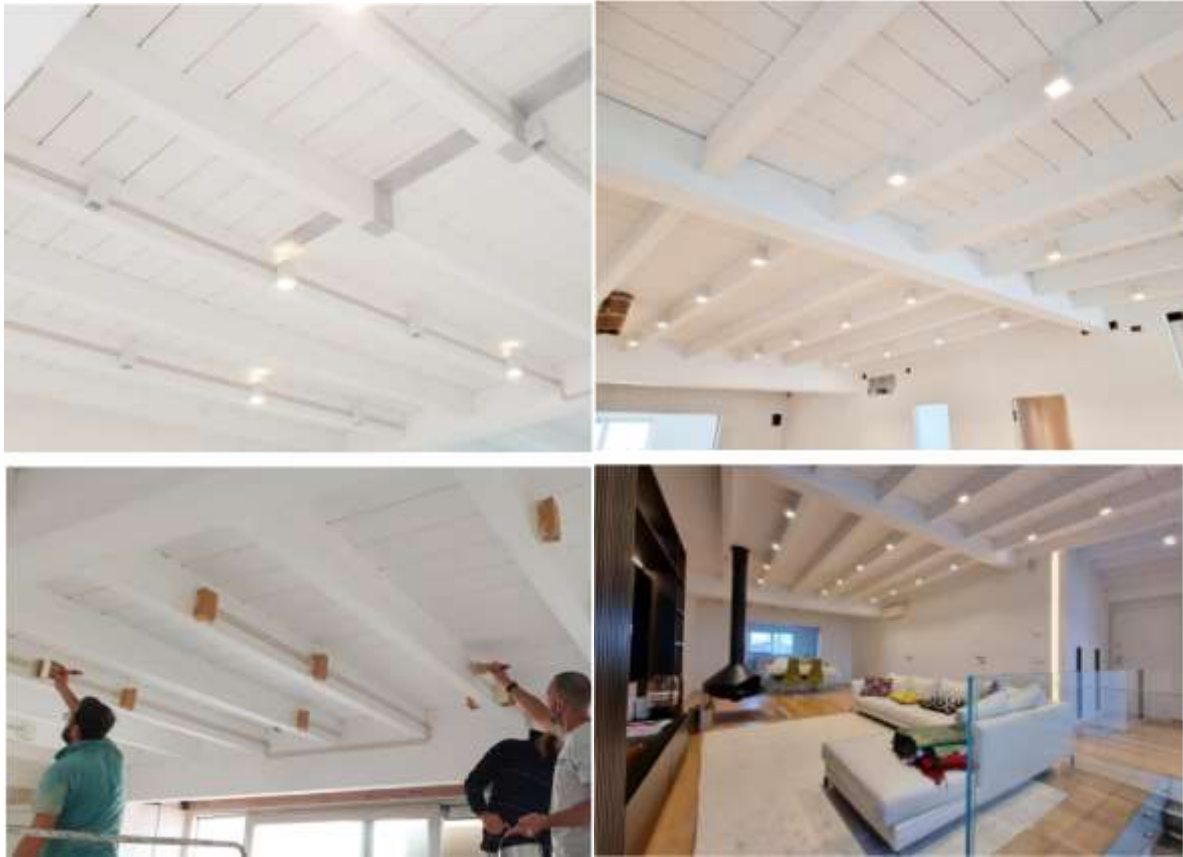
Figure 22: Construction of a ceiling lighting system for a private apartment with NM4BT05 electrical tape.
